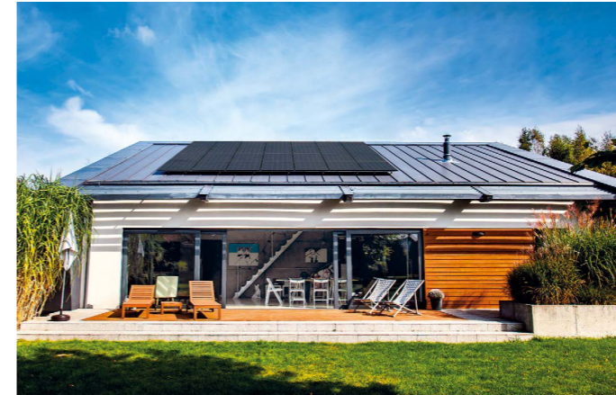
JUNONY, POLAND 6.4 kWp
